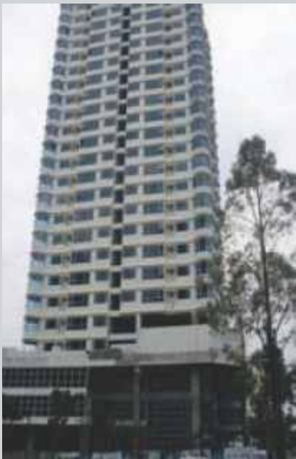
Seibu Tower Project
